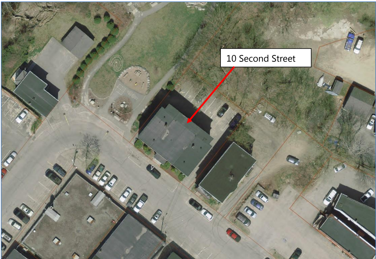
23 Broad St. Aerial View
